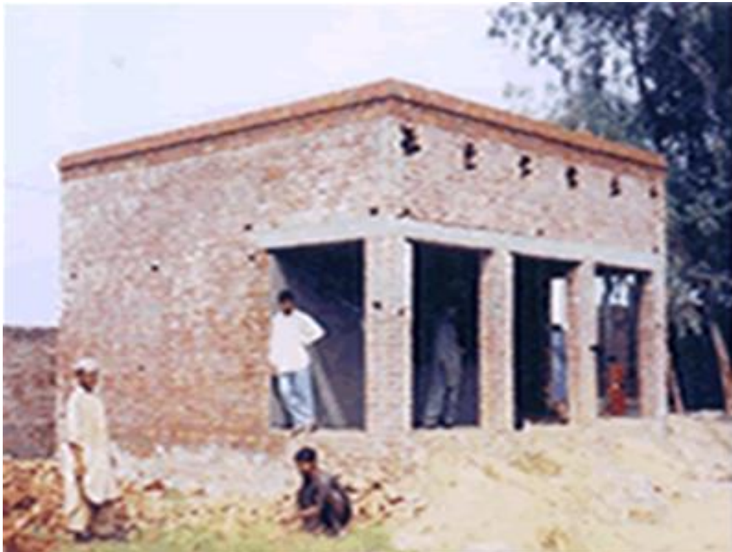
Construction Progress in 2001
