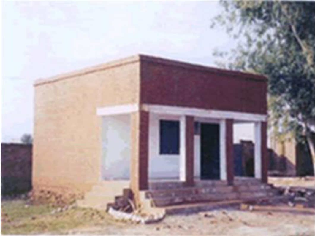
Construction Progress in 2001
