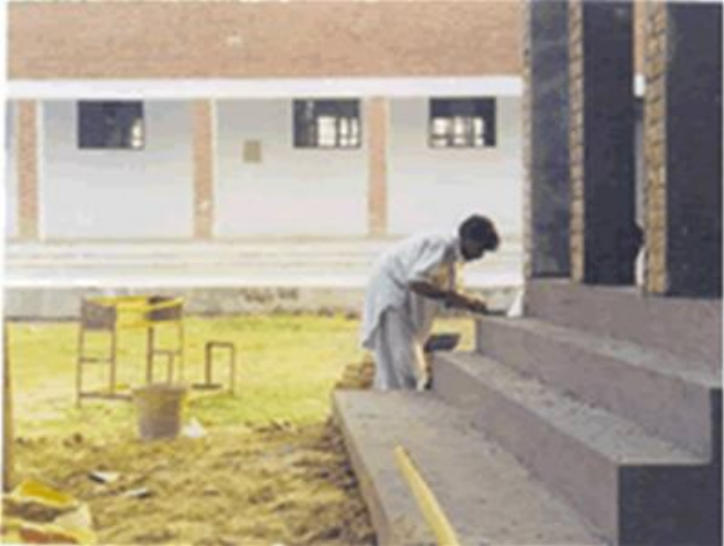
Construction Progress in 2001
