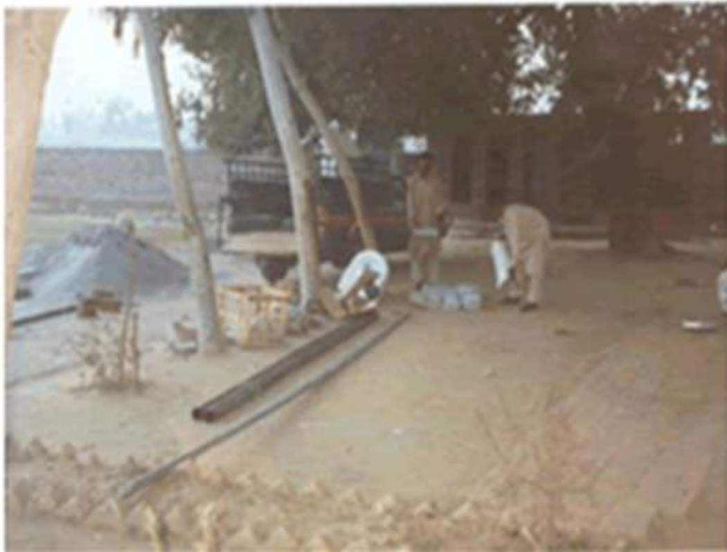
Construction Progress in 2000
