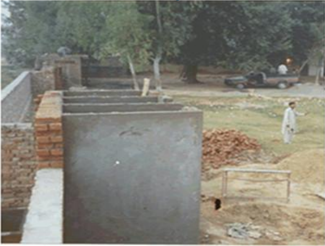
Work underway to construct bathrooms in 2000
