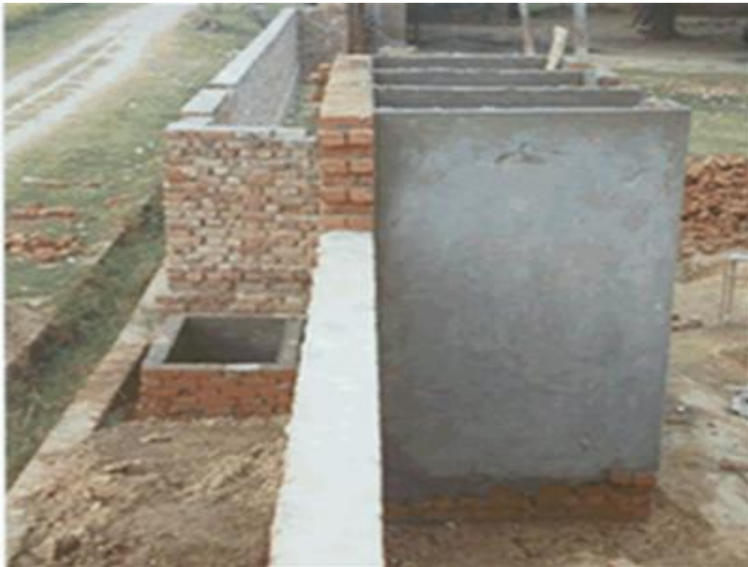
Work underway to construct bathrooms in 2000
