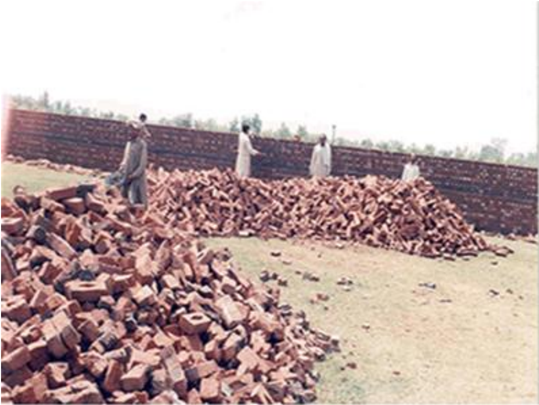
Construction Progress in 2000
