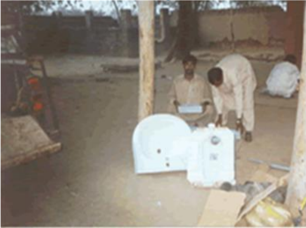
Construction Progress in 2000
