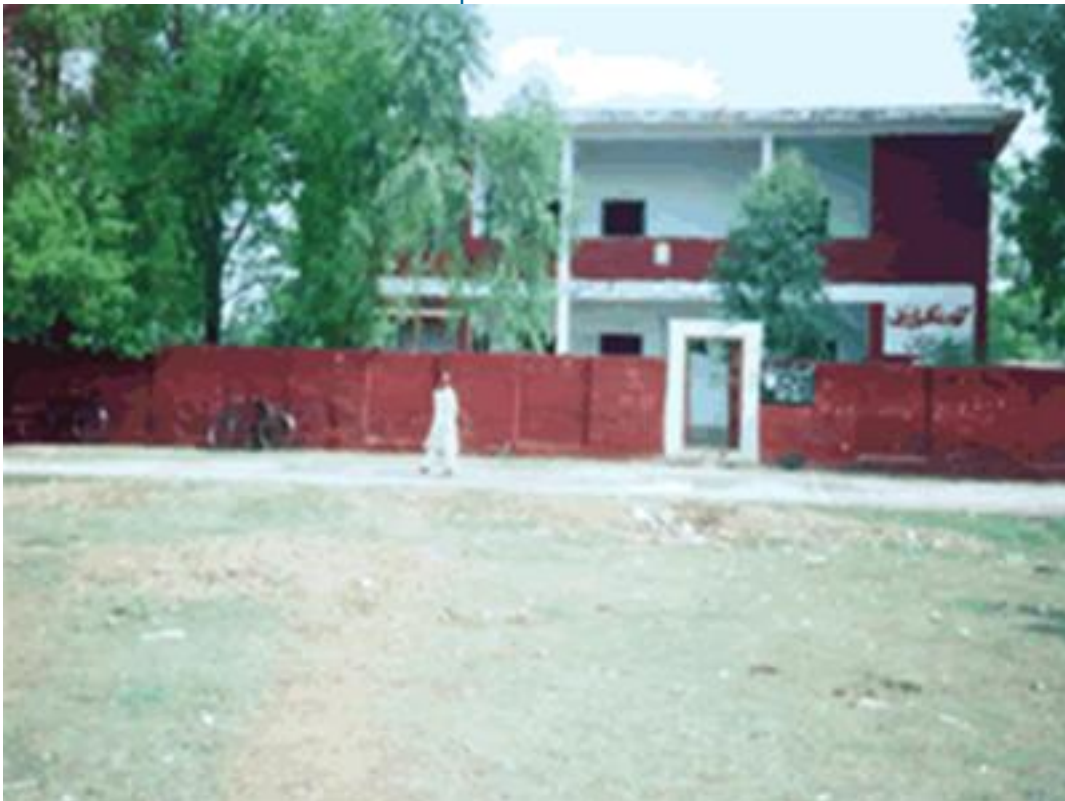
Front view of school
